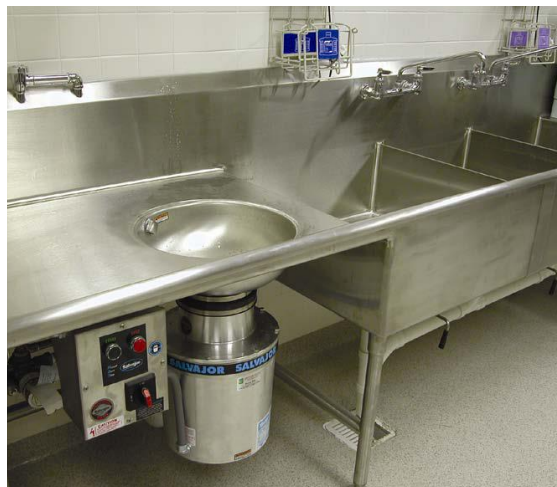
Figure 2: An example of a commercial food waste disposer (NYC DEP 2008)
